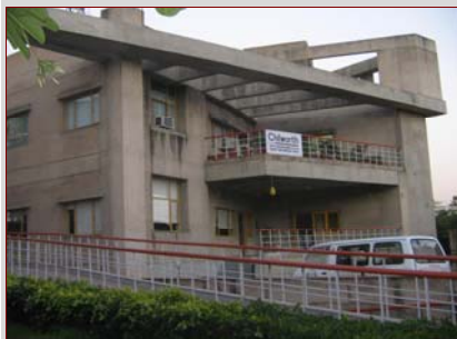
Chilworth India HQ at New Delhi
